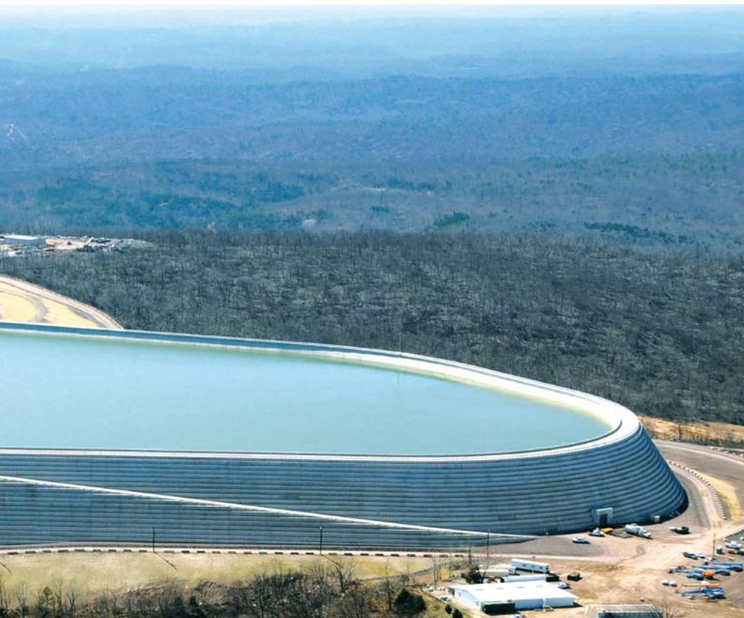
the existing rhyolite rock-fill dam, repairing the base foundation, and placing RCC and formed conventional concrete back into the proximity of the original footprint of the reservoir. All aggregate used in the RCC was recycled from the original structure and crushed on-site.
