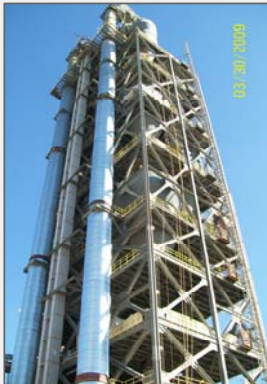
Pre-heater tower and stack
