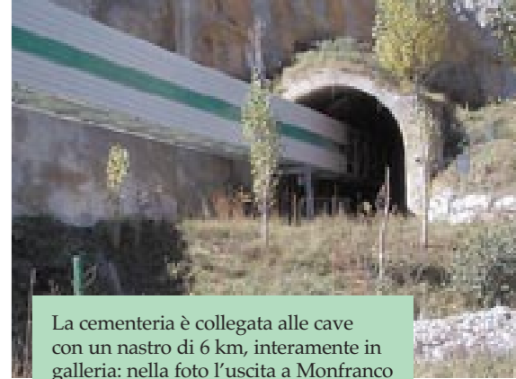
The plant is connected to quarries by a 6-km conveyor belt, inside a tunnel: in the picture the belt at Monfranco quarry
